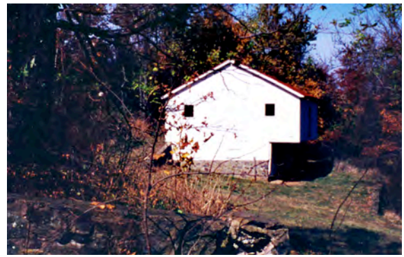
Figure 15. Snead Farm stone house foundation and barn (Shenandoah National Park), 2001.
